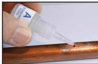
Step 1: After sanding, apply BONDING FLUID (A) to repair area
